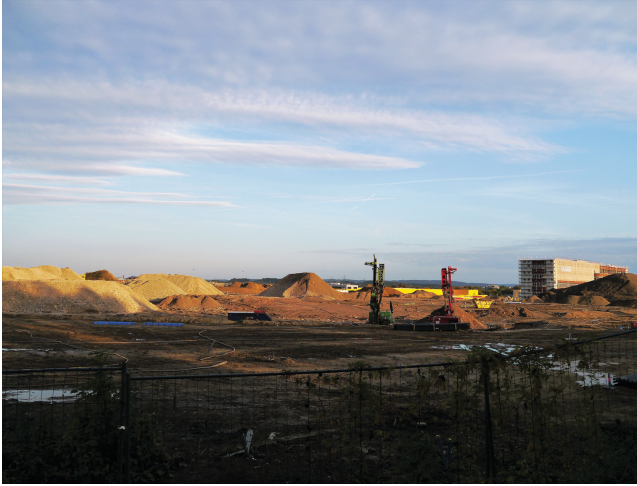
Figure 4.6 The site of Mark 51°7 in October 2019 (the former Opel admin building is on the right).
