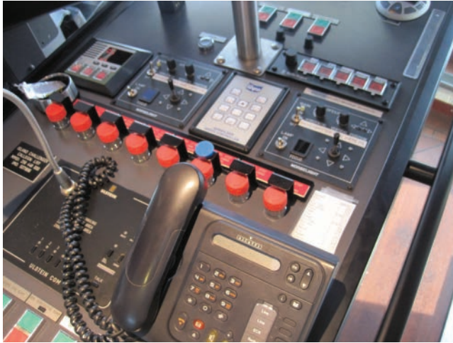
FIGURE 9.1 Whiteboard magnet to visualize the active emergency stop button.
